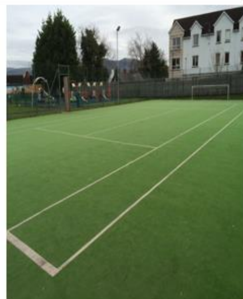
Refurbished Astro Turf.
